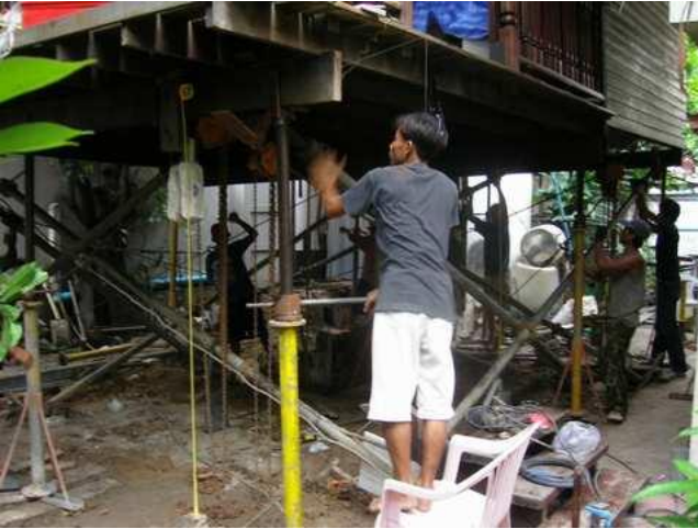
Local technology...Lifting up the house
