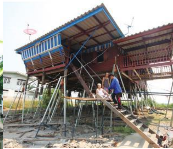
Local technology...Lifting up the house
