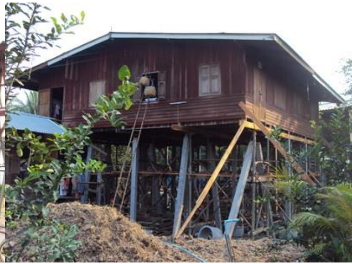
Local technology...Lifting up the house
